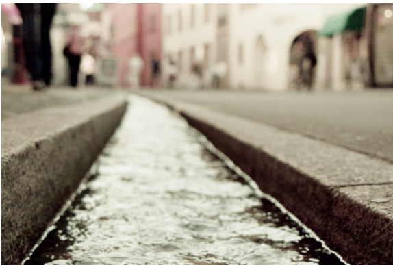
“Venice for your feet”: Freiburg has an unique system of small canals (called Bächle) that run throughout the centre. During the summer, the running water provides natural cooling of the air and offers a pleasant gurgling sound. © Rob Faulkner
